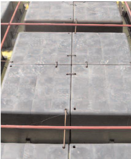
The system is easily installed. The plumbing is brought up through the WAFFLEBOXES with rebar reinforcement. The slab setup and pour is a two-day or less process, eliminating trenching and reducing soil preparation by providing less over-excavation and re-compaction, reducing building cycle-time.
