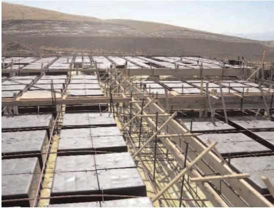
The WAFFLEMAT foundation forming system creates a post-tensioned foundation especially for expansive soils. It offers the ease of constructability of a Uniform Thickness Foundation, along with the effectiveness of a Ribbed Foundation.
