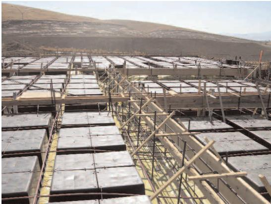
The WAFFLEMAT foundation forming system creates a post-tensioned foundation especially for expansive soils. It offers the ease of constructability of a Uniform Thickness Foundation, along with the efficiency of a Ribbed Foundation.
